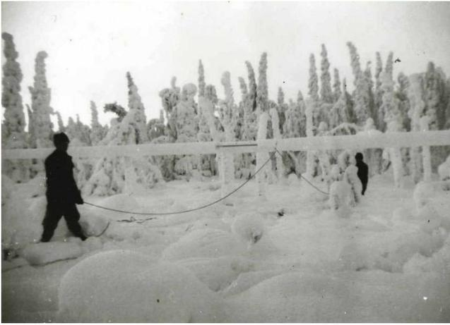
Fig. 3 Picture demonstrating an icing event including dry snow in January 1951 in near Slagnäs, Northern Sweden. Provided by Svenska kraftnät.
