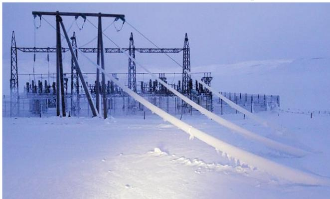
Fig. 15 Ice diameter is much less at suspension points than in the middle of the span and close to the ground.
