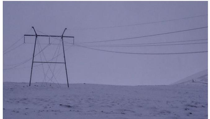
Fig. 13 Icing on the last span of TR 1. Earth wire sagged below conductors after the ice was removed from the conductors. The icing on earth wire is ~ 9 kg/m.
