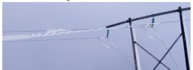
Fig. 19 Spiral form of icing due to sliding of accumulation.
