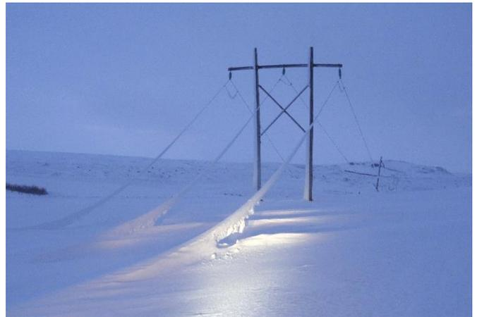
Fig. 16 Icing on KS1. When the conductors come close to the earth, there is an extra accretion because of drifting snow.
