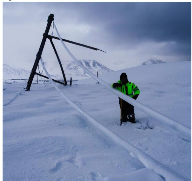
Fig. 7 Icing on conductors next to failed tower.
