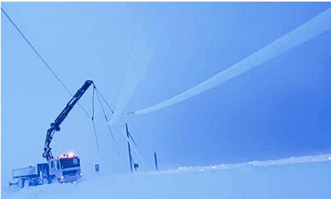
Fig. 10 Icing at Hámundarstaðaháls, elevation ~70 m a.s.l. Crane holding conductors above road crossing after failure.
