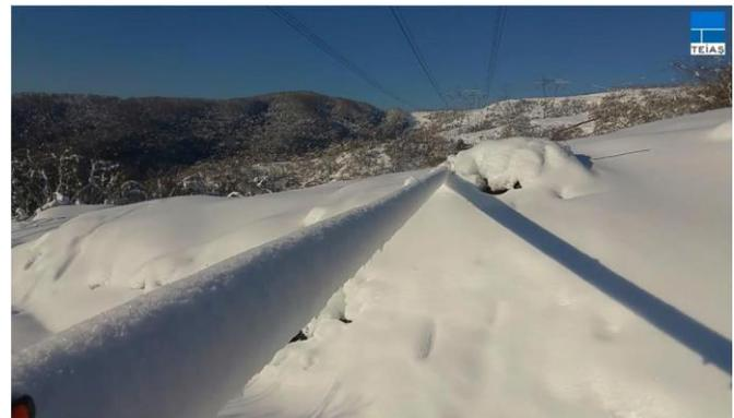
Fig. 2 Wet snow sleeve on a 170 kV line in the Marmara region, December 2016.
