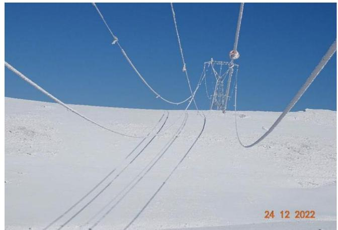
Fig. 1 Rime icing on the 170 kV line in the North-east region, December 2022.
